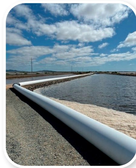
Cheetham built a new launder at Port Alma to protect our operations from the impact of accelerating river creek erosion.
